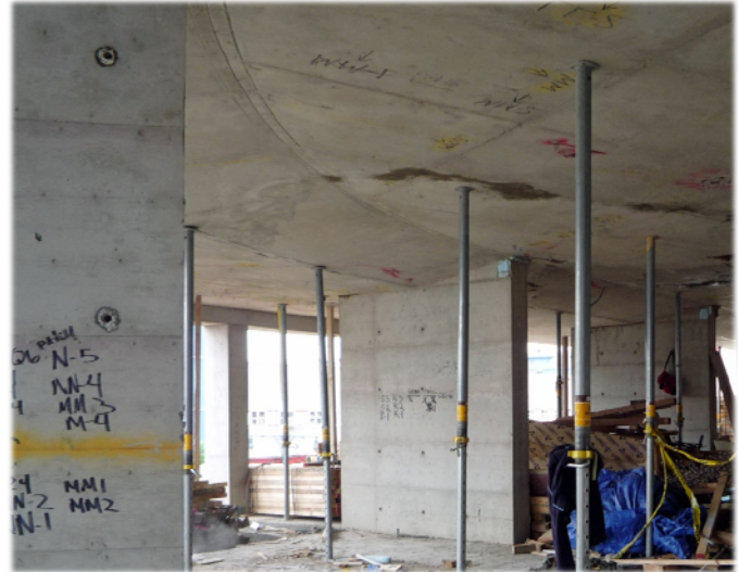
Figure D2: View of thickened slab
