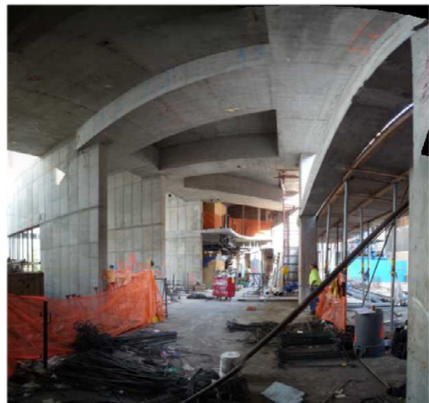
Figure 10: 3rd Floor transfer beams
