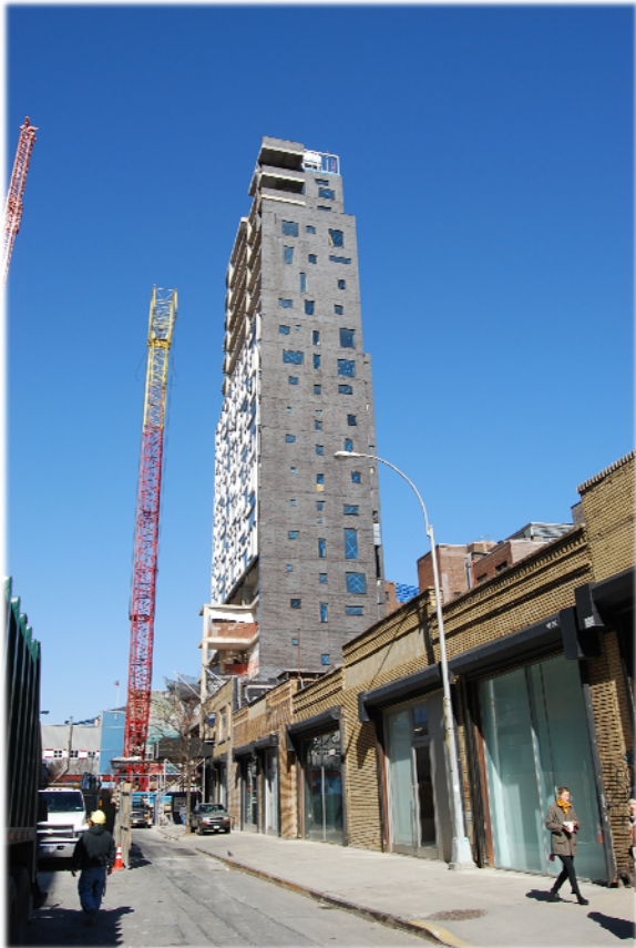
Figure D1: View looking west of the dark gray brick facade
