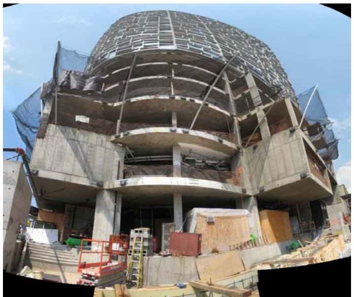
Figure 13: Photo showing portion of cantilevered balcony system
